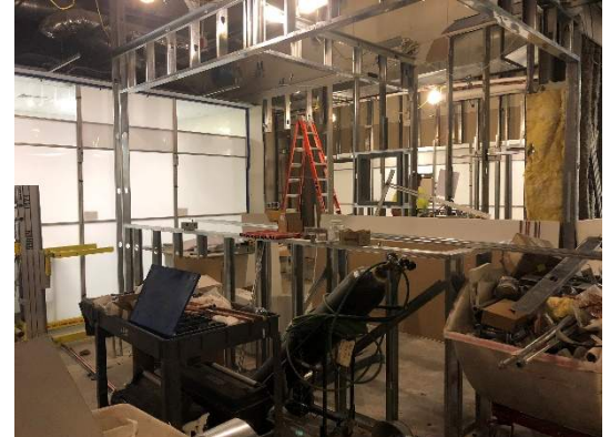
A few photos peering into the new ER Nurse Station. Stud walls have been installed and MEP rough ins are nearly complete! The space will be ready for drywall installation soon.
