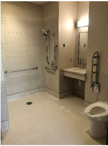
The photos above show the progress update on the upper level Clinic / Med Surge addition. The bathrooms have ceramic tile installed along with fixtures and accessories, millwork and wall protection has been installed, and within the patient rooms the 3form wheat panels are being installed within the headwall units!
