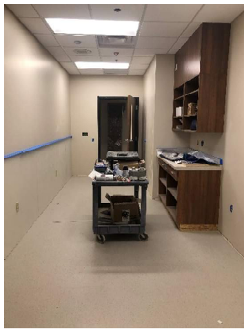
The photos above show the progress update on the upper level Clinic / Med Surge addition. The bathrooms have ceramic tile installed along with fixtures and accessories, millwork and wall protection has been installed, and within the patient rooms the 3form wheat panels are being installed within the headwall units!
