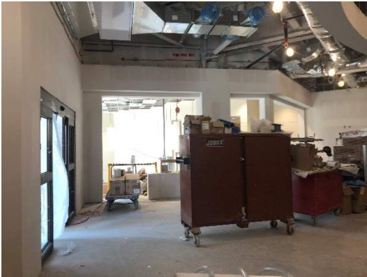
The photos above depict the new Outpatient Clinic! The walls have received their first coat of paint and the millwork has been installed. You can see the handles on the millwork are put on backwards. This is to protect them while construction is still ongoing. When most of the trades are complete in the space, the handles will be installed on the front size.
