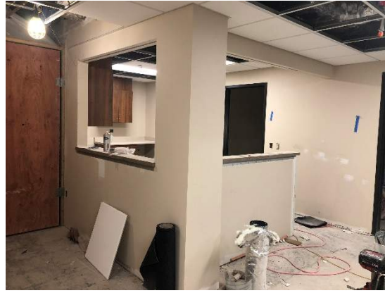
The photos above depict the new Outpatient Clinic! The walls have received their first coat of paint and the millwork has been installed. You can see the handles on the millwork are put on backwards. This is to protect them while construction is still ongoing. When most of the trades are complete in the space, the handles will be installed on the front size.
