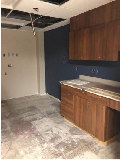
The photos above depict the new Outpatient Clinic! The walls have received their first coat of paint and the millwork has been installed. You can see the handles on the millwork are put on backwards. This is to protect them while construction is still ongoing. When most of the trades are complete in the space, the handles will be installed on the front size.
